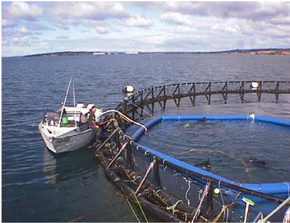
Figure 12. Deployment of the enclosure (in its 3panel 36 metre configuration) and gas ring (being positioned by divers) from the "Toro."
