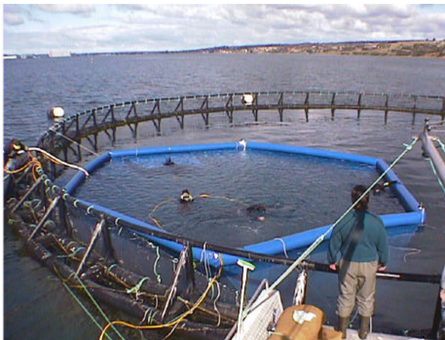
Figure 13. Full liner deployed.
